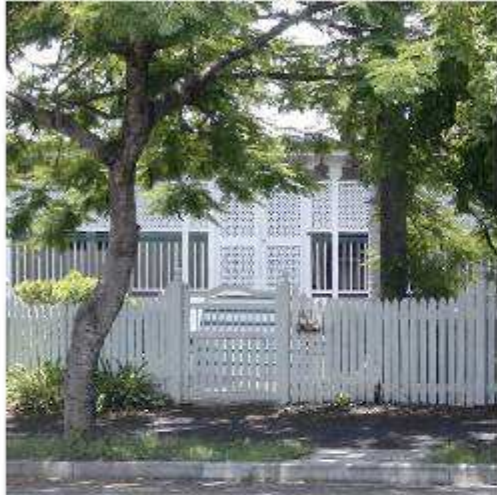
Rich layering of entrance transition and occupied verandah areas of houses
