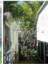
Spaces between buildings look into treed back gardens
